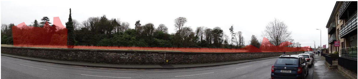
Plate 19. Panoramic view of the site along Academy Street (southern section)
