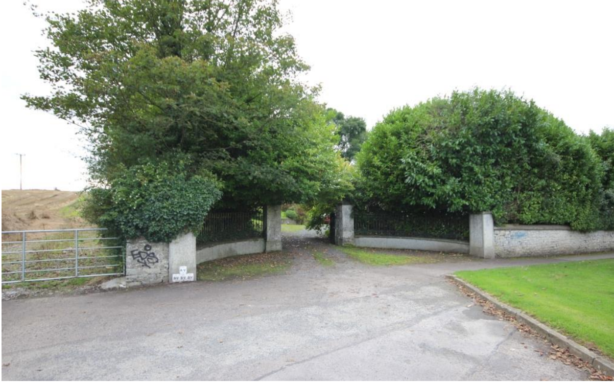
Plate 13.2: View of the former southern entrance to Belmont House (on the Dublin Road). This now forms the entrance to a modern private residence; the driveway that led towards Belmont House is no longer in use and extends into the proposed development site.
