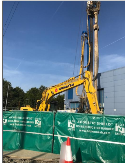
Acoustic blankets screening piling and excavations
