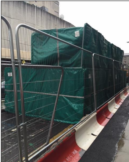
Double height acoustic blanket enclosure
